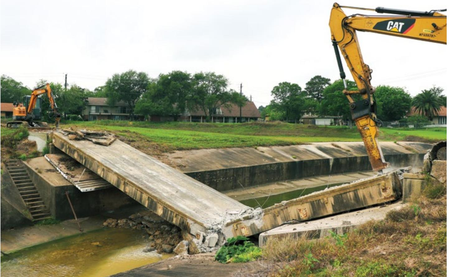
The ends of the bridge were cut using a Pentrunder 8-20HF wall saw.
